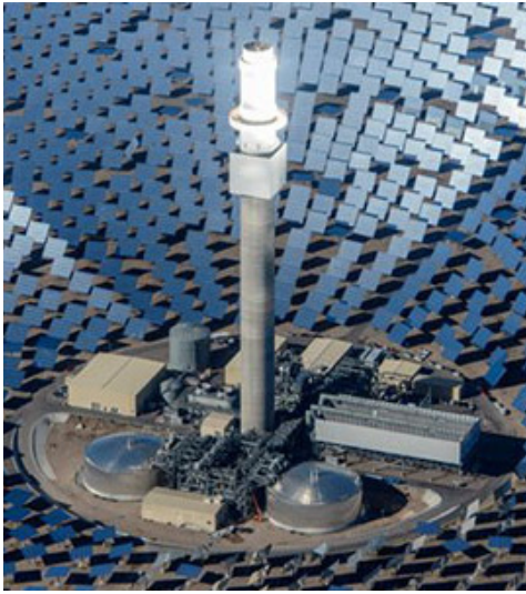
The Crescent Dunes solar storage project near Tonopah, Nev., concentrates sunlight to heat molten salt to 1000 degrees. | Solar Reserve
